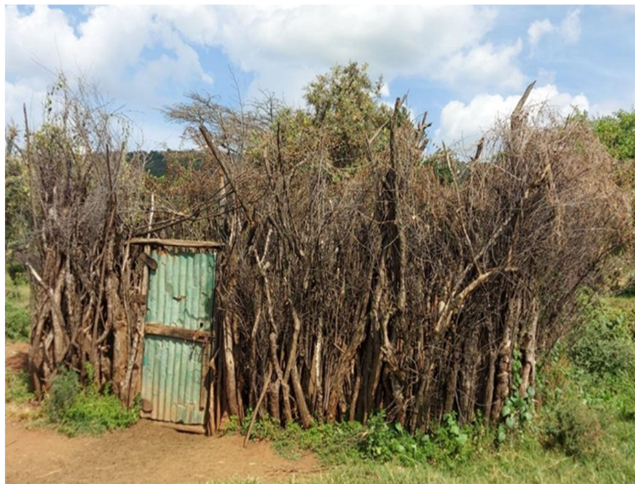
Figure A2. Traditional Kraal build using twigs and tree branches.
